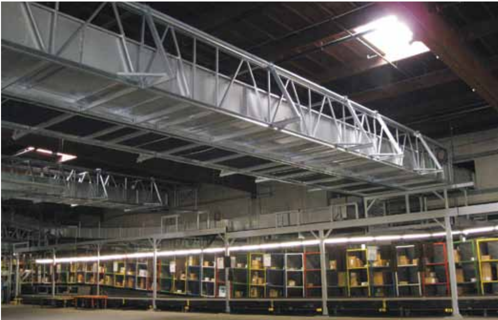
Figure 1: TrusSteel CFS Truss Bridge over drive-thru bay.
